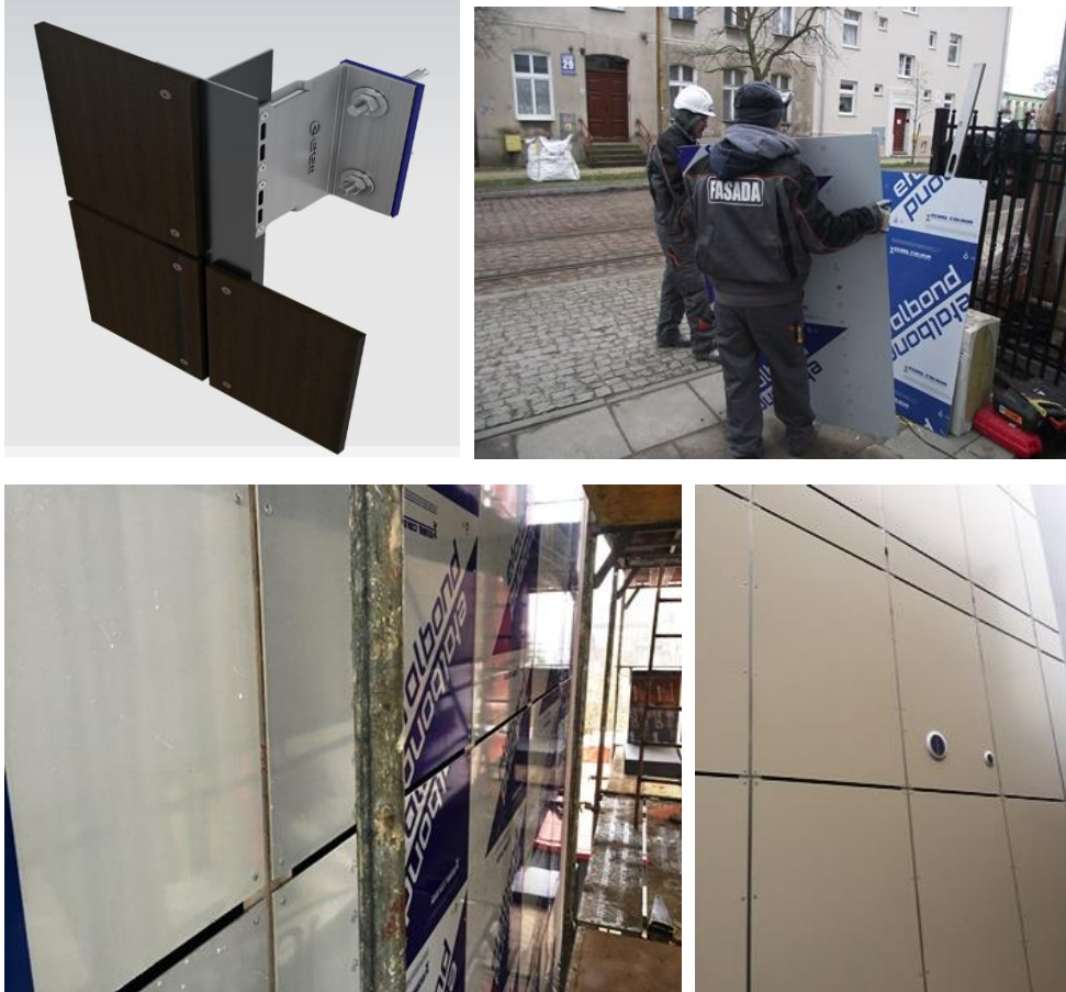
Figure 9: Rivet fixing system used during demonstrations.
